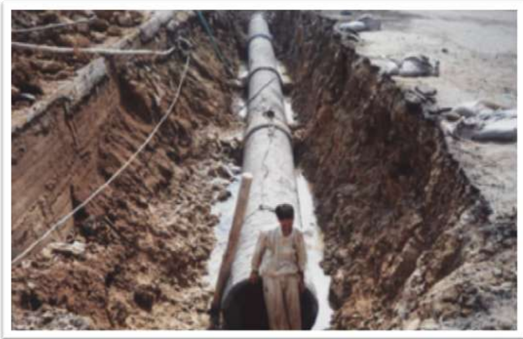
LAYING OF 33" DIA PRCC PIPES AT GULISTAN-E-JAUHAR
