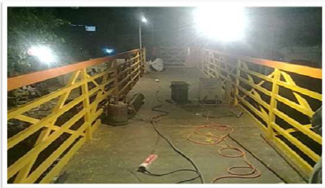
FABRICATION OF OVERHEAD PEDESTRIAN BRIDGE IS IN PROGRESS
