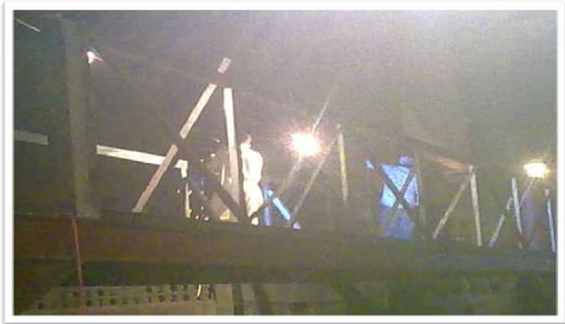
WELDING OF CHANNELS AT NIGHT FOR PEDESTRIAN BRIDGE IS IN PROGRESS
