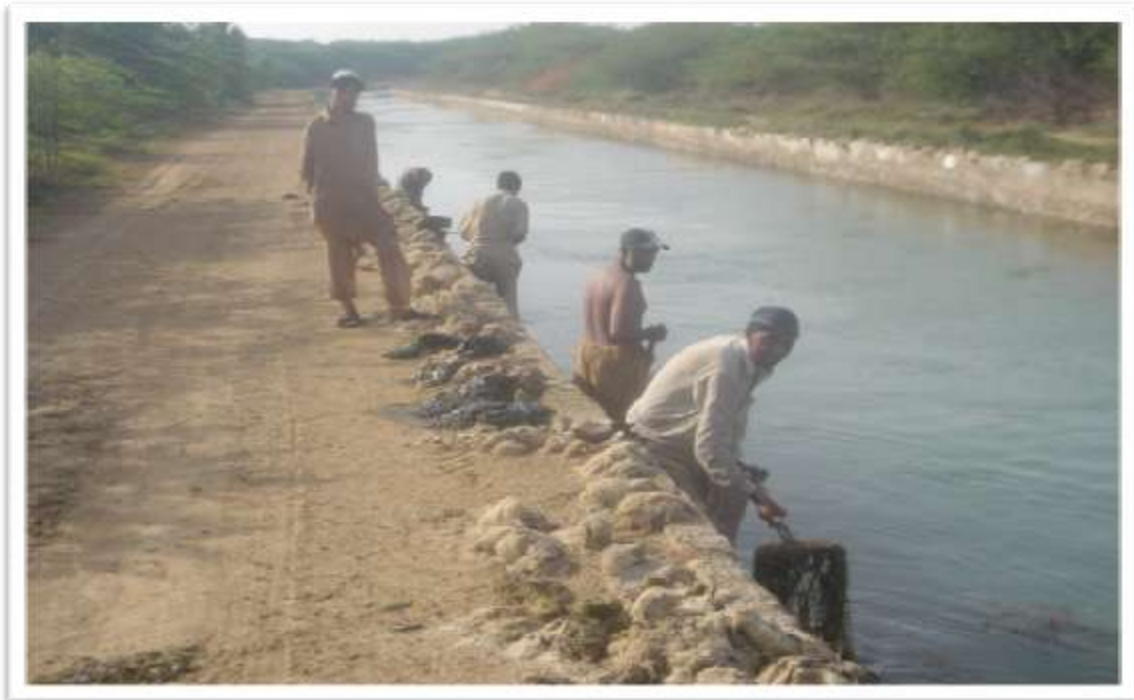
DESILTING OF HUB CANAL BY LABORS
