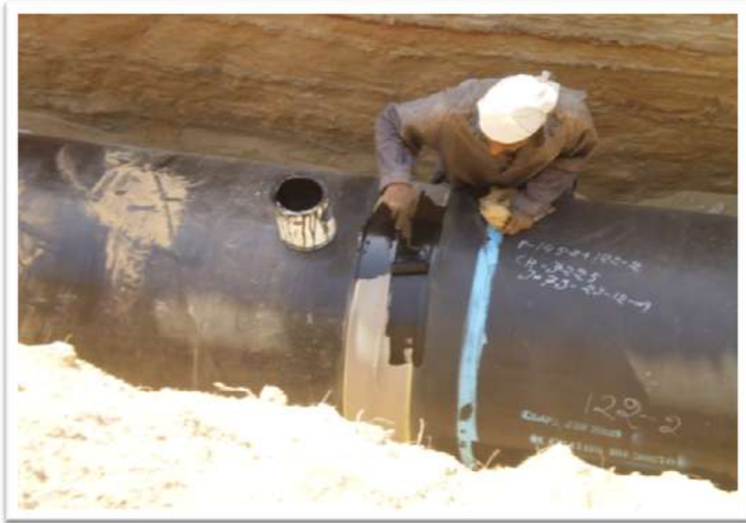
APPLICATION OF PRIMER AT PIPE JOINT
