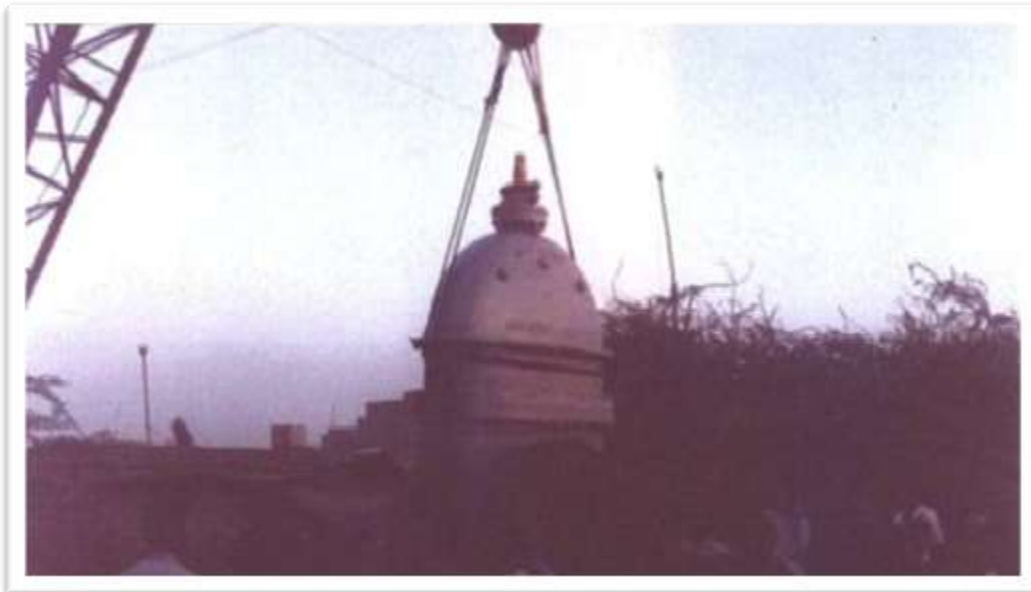
REPLACEMENT OF SLUICE VALVE AT SURJANI TOWN
