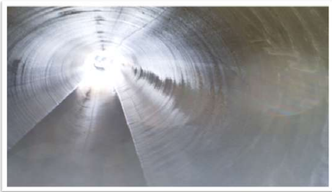
INTERNAL FACE OF PIPE AFTER PROCESS OF INTERNAL LINING
