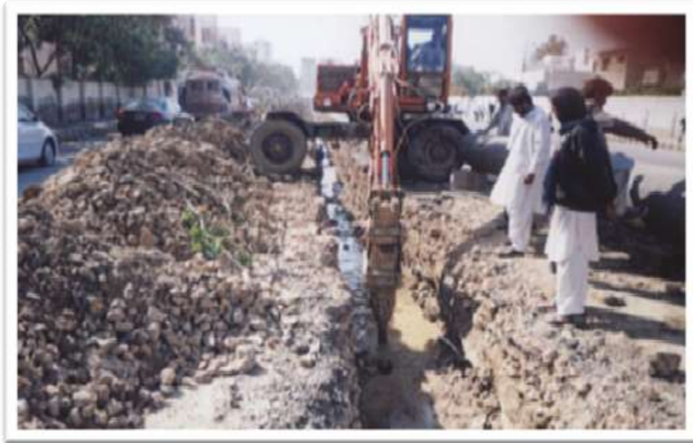
EXCAVATION IN PROGRESS AT SADDAR TOWN
