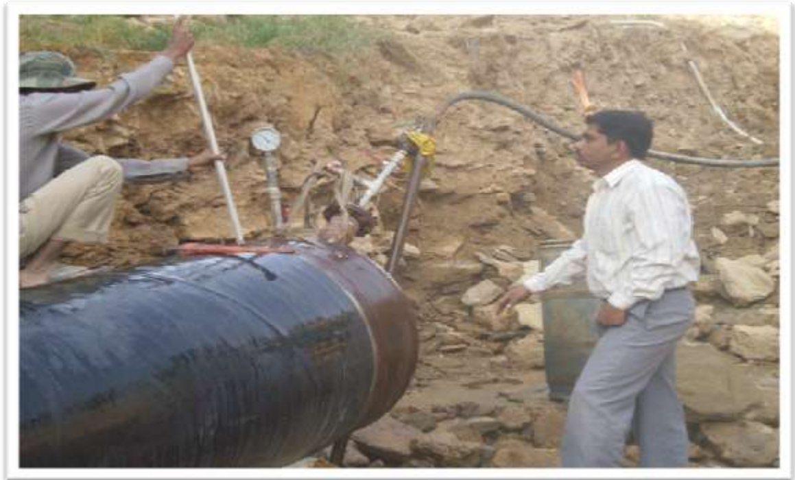
HYDROSTATIC TEST IS IN PROGRESS AT PIPRI WATER SUPPLY PROJECT
