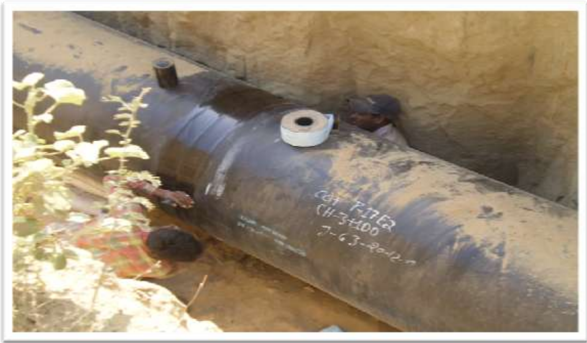
PE COATING OF MS PIPES IS IN PROGRESS
