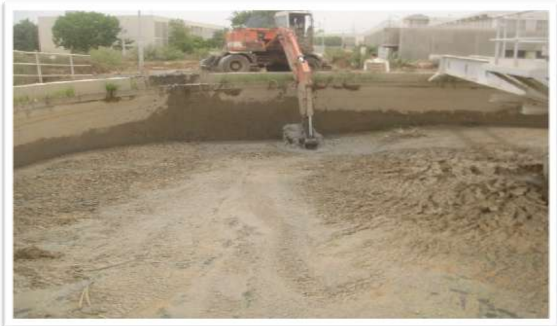
SILT CLEANING AT NEK FILTER PLANT IS IN PROGRESS
