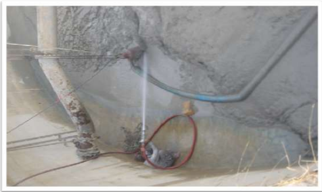
PRESSURE CLEANING AND SUBMERSIBLE PUMP IS IN PROGRESS
