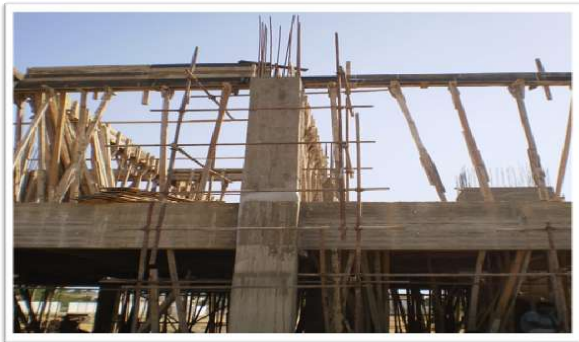
CONSTRUCTION OF HOUSING FACILITIES FOR CDGK
