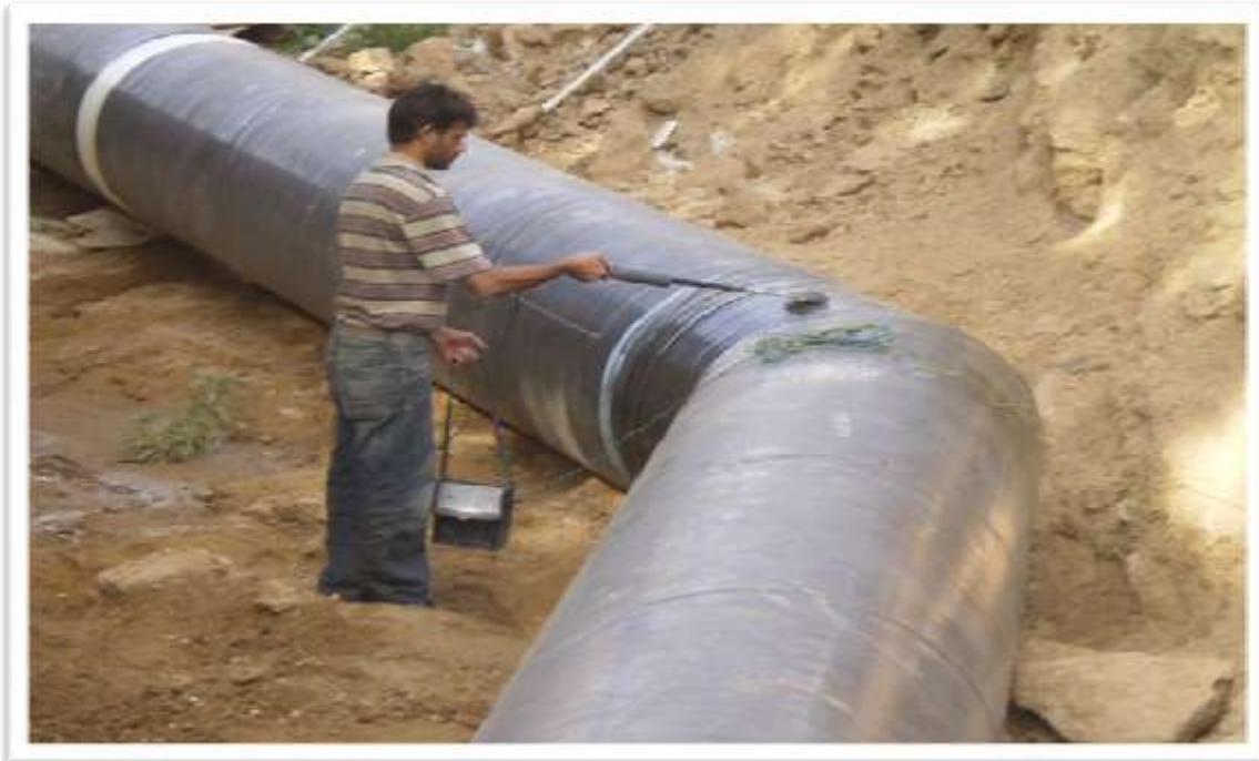
HOLIDAY DETECTION TEST IS IN PROGRESS
