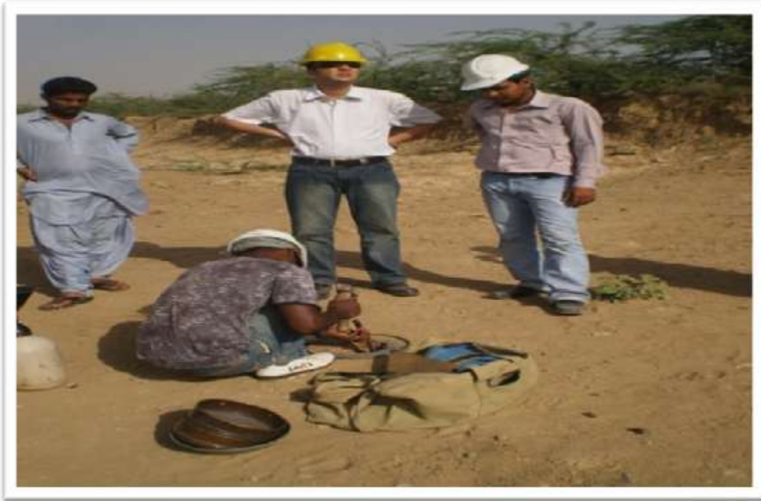
FIELD DENSITY TEST IS IN PROGRESS AT PIPRI WATER SUPPLY PROJECT
