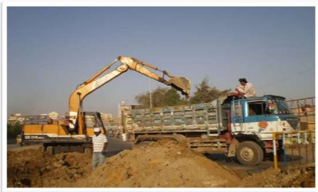
DISPOSAL OF EXCAVATED UNUSED MATERIAL FROM SITE
