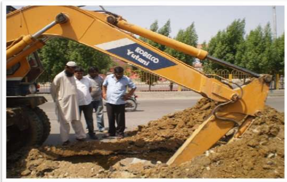
EXCAVATION IS IN PROGRESS AT GULSHAN-E-IQBAL NEAR SAFARI PARK
