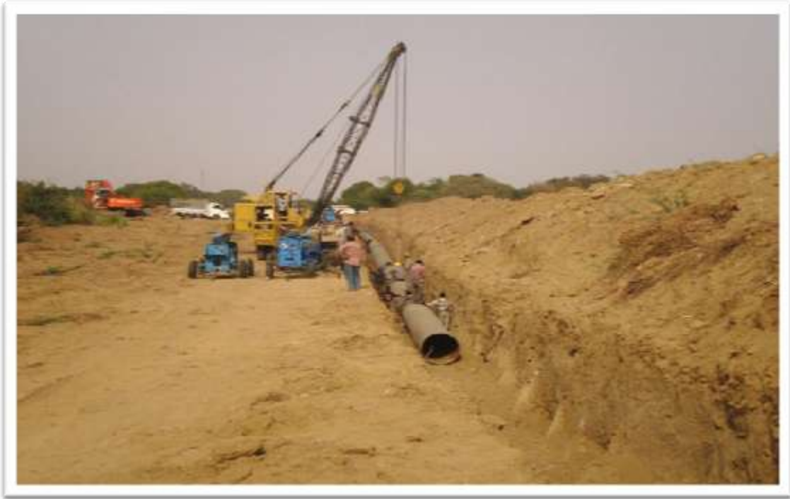
PIPE LAYING ACTIVITY IS IN PROGRESS BY CRANE
