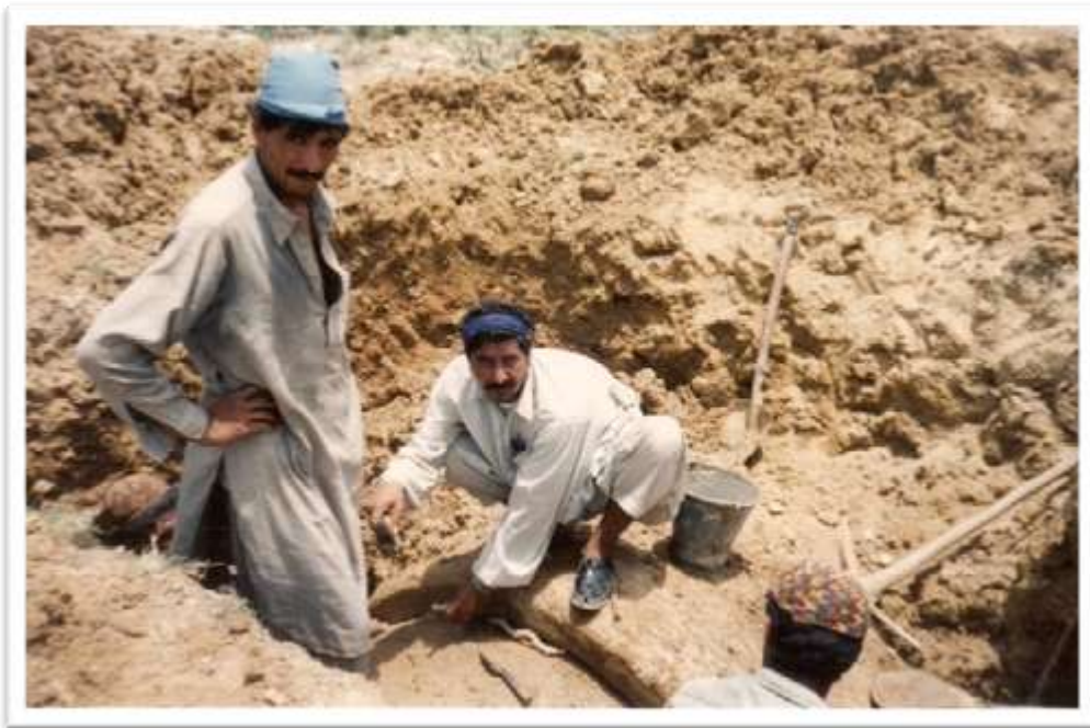
REPAIR WORKS ON LEAKAGES OF 54" DIA PRCC PIPELINE AT SCHEME 33
