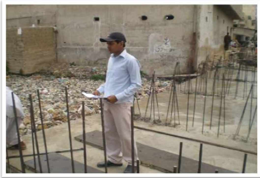
OUR ENGINEER'S INSPECTION OF BASE SLAB OF CULVERT
