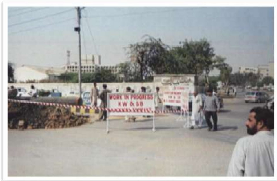
EMERGENCY WORK AT SADDAR TOWN ROAD
