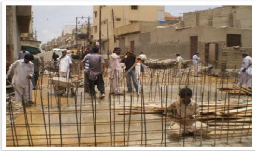
REBAR FIXING & FORMWORK FOR THE CONSTRUCTION OF NORTH NAZIMABAD CULVERT
