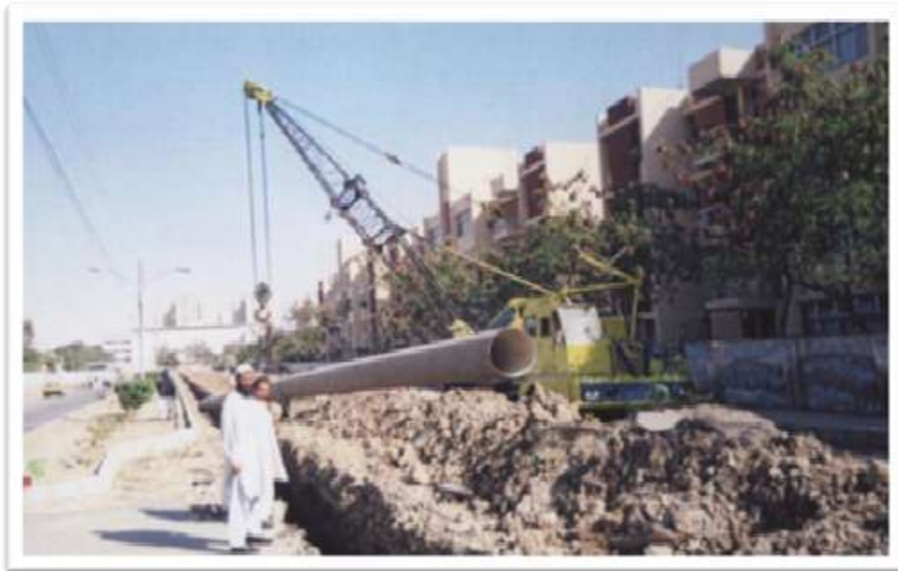
LAYING OF 24" DIA MS PIPELINE AT LILLY BRIDGE, SADDAR TOWN
