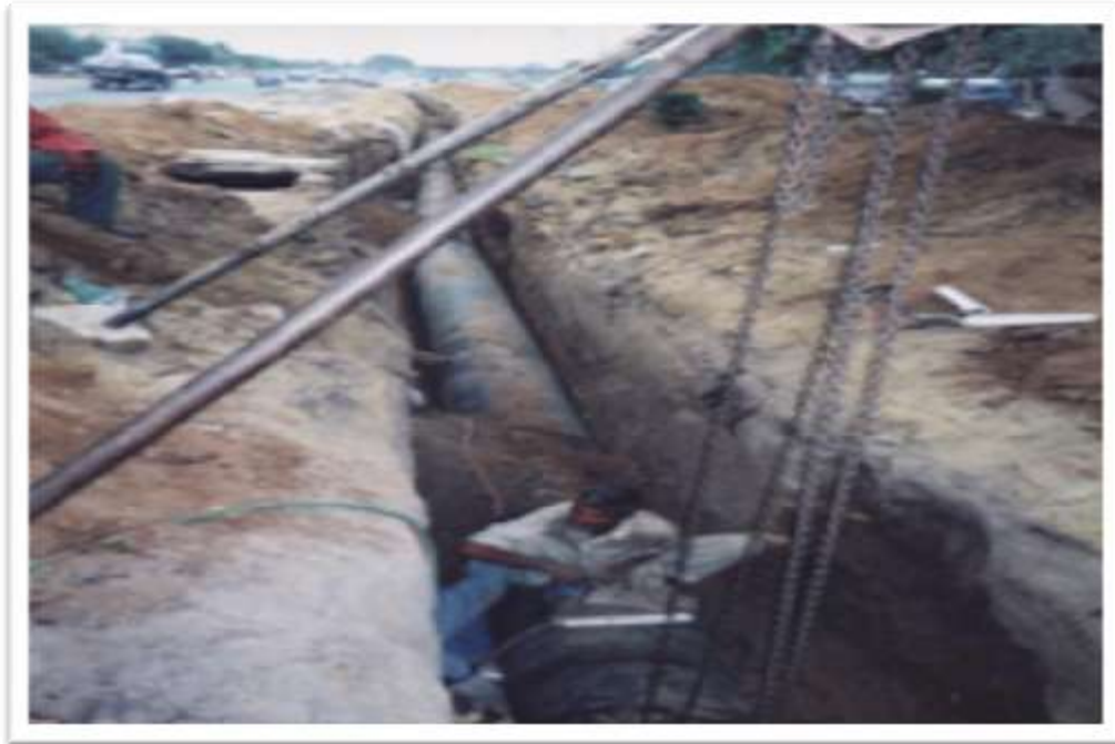
LAYING OF 33" DIA PRCC PIPES AT GULISTAN-E-JAUHAR
