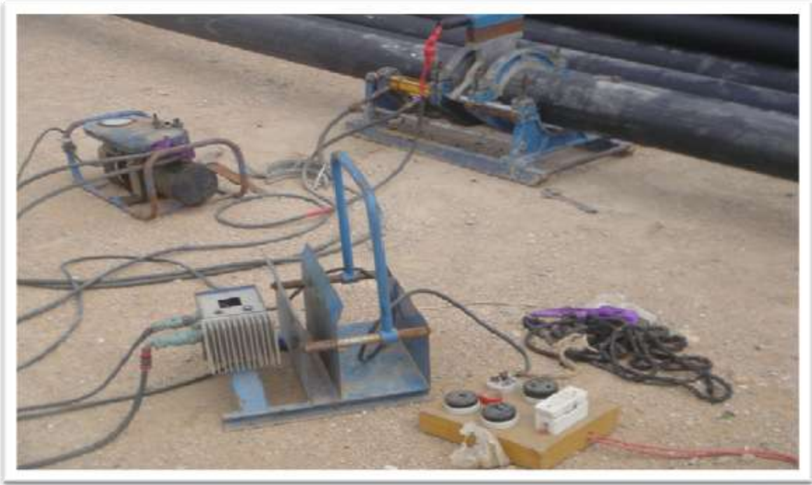
JOINTING OF PE PIPE BY FUSION PROCESS
