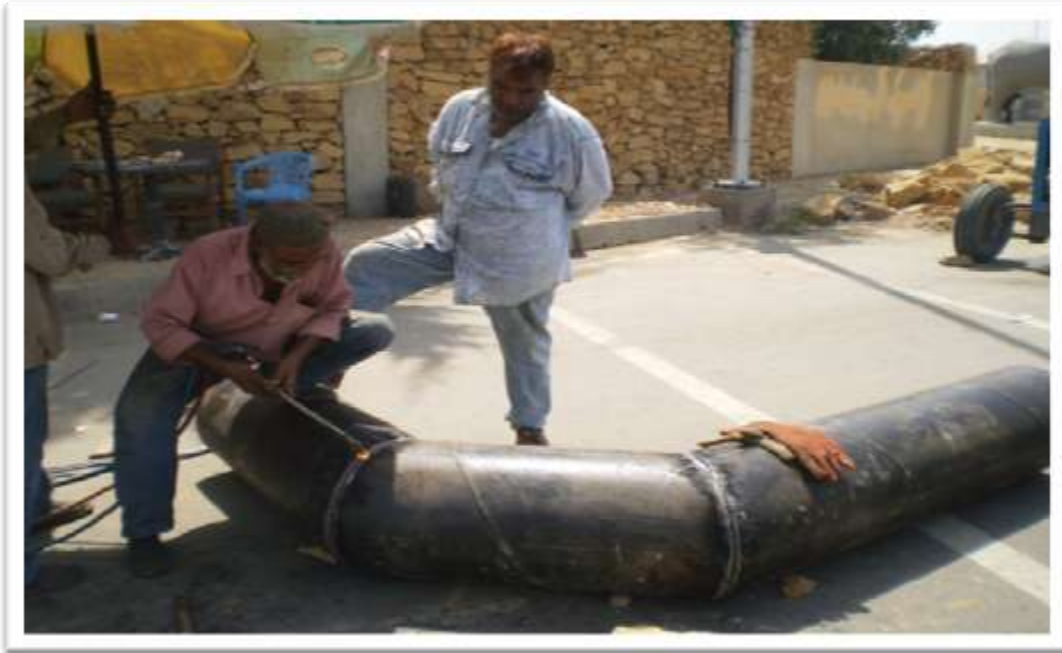
FABRICATION OF MS BENDS IN PROGRESS
