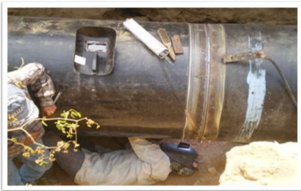
WELDING OF JOINTS IS IN PROGRESS
