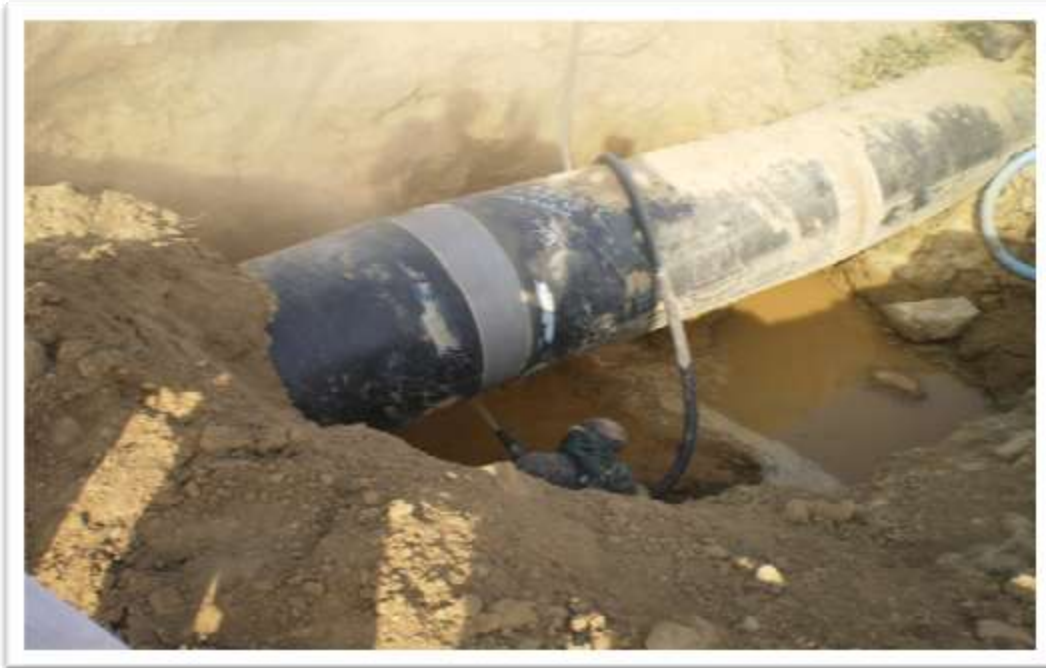
SAND BLASTING OF PIPE IS IN PROGRESS
