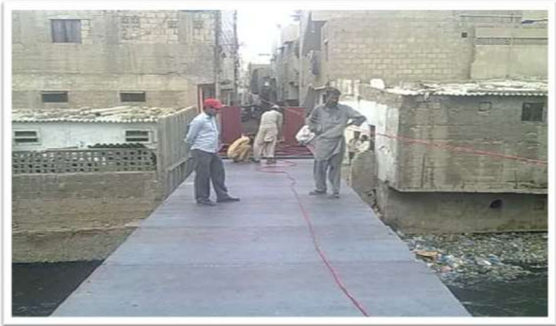
FIXING OF CHECKER PLATE FOR PEDESTRIAN BRIDGE IS IN PROGRESS
