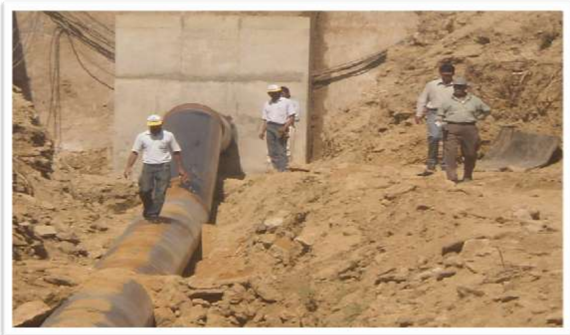
INSPECTION BY CLIENT AND CONSULTANT AFTER CONSTRUCTION OF INTERCONNECTION CHAMBER
