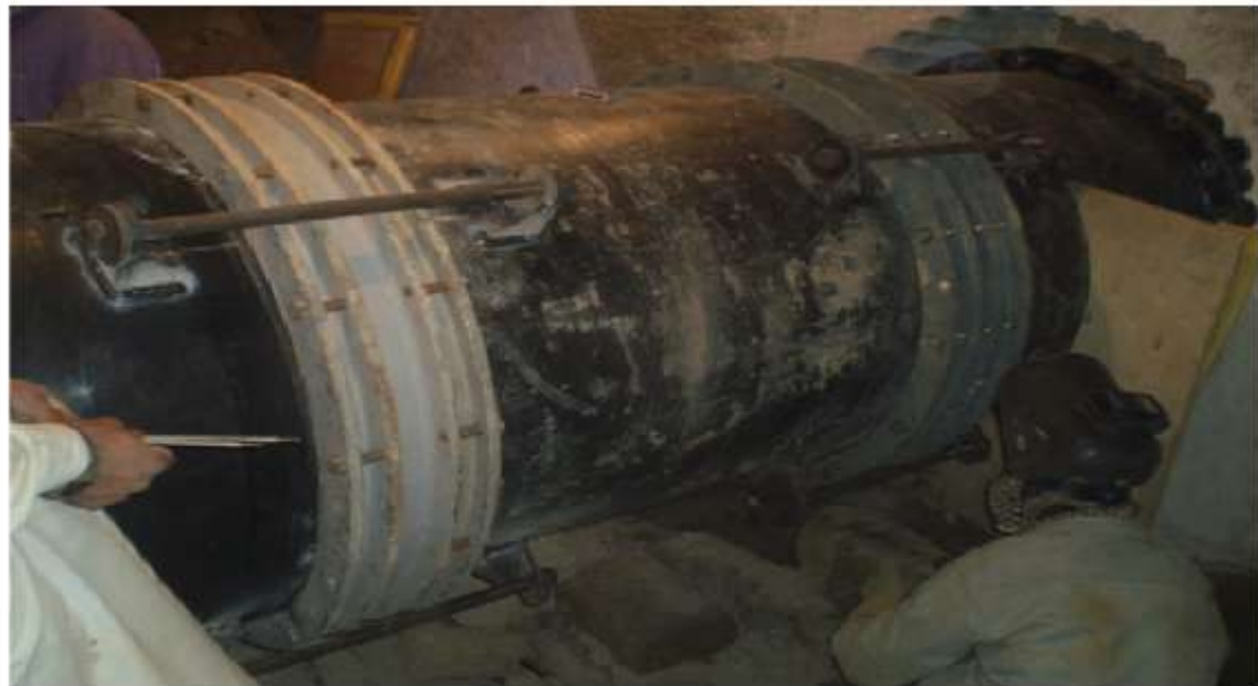
FIXING OF SPOOL AT INTERCONNECTION AFTER CORE CONCRETE CUTTING OF RESERVOIR
