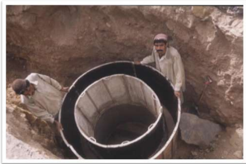
CONSTRUCTION OF SEWER AT GULISTAN-E-JAUHAR
