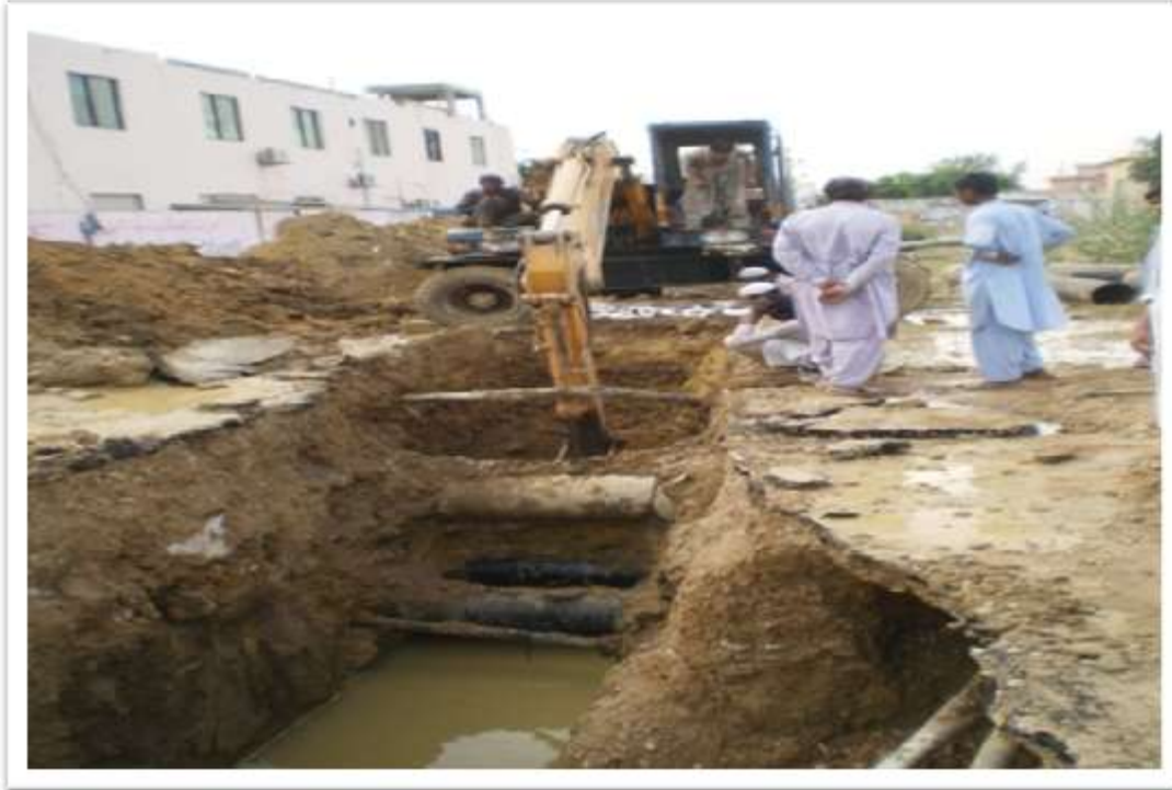
EXCAVATION OF TRENCH NEAR SAFARI PARK
