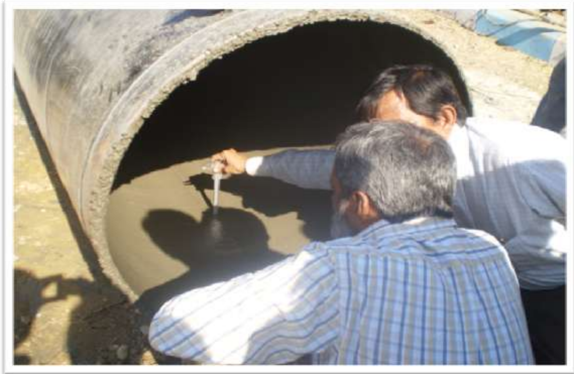
INSPECTION OF INTERNAL CEMENT MORTAR LINING BY THE CONSULTANT
