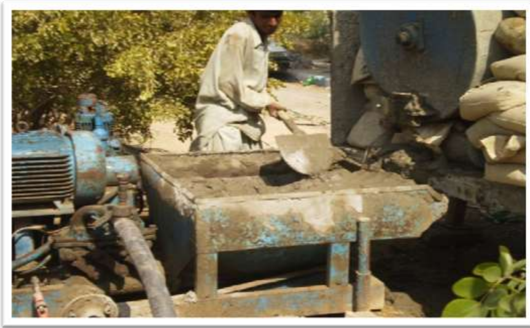
MORTAR MIXING FOR INTERNAL LINING IS IN PROGRESS
