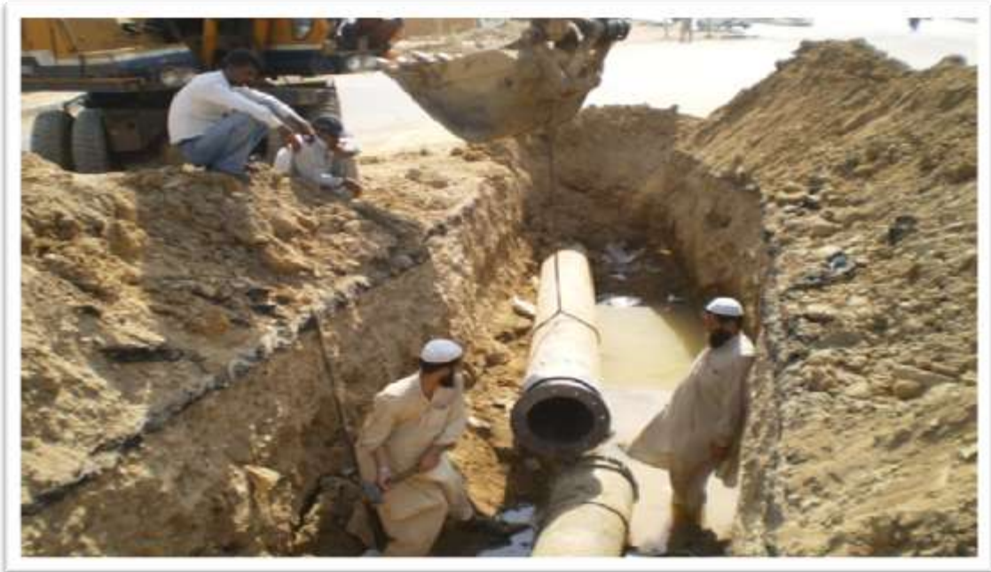
CONNECTION OF PE PIPE TO MS PIPE NEAR SAFARI PARK
