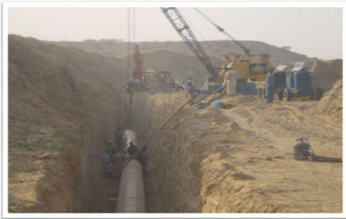
PIPE LAYING ACTIVITY IS IN PROGRESS AT SITE
