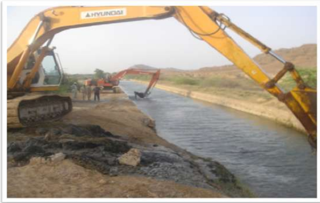
DESILTING OF HUB CANAL BY LONG STICK EXCAVATORS
