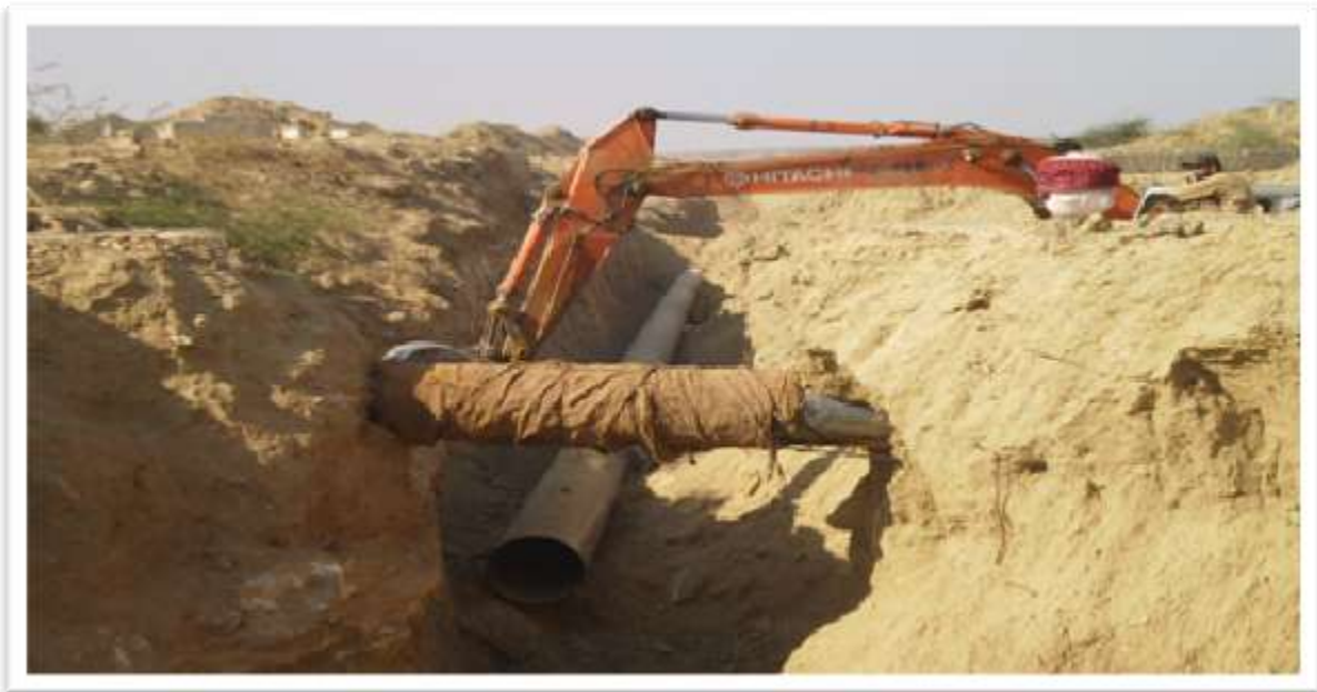
EXCAVATION IS IN PROGRESS FOR MS PIPES
