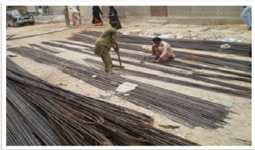
CUTTING OF STEEL FOR CONSTRUCTION OF NORTH NAZIMABAD TOWN CULVERT
