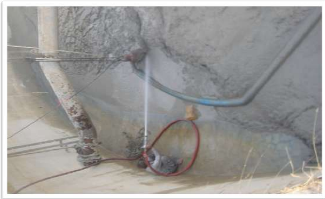
PRESSURE DESILTING OF RESERVOIR BY SUBMERSIBLE PUMP
