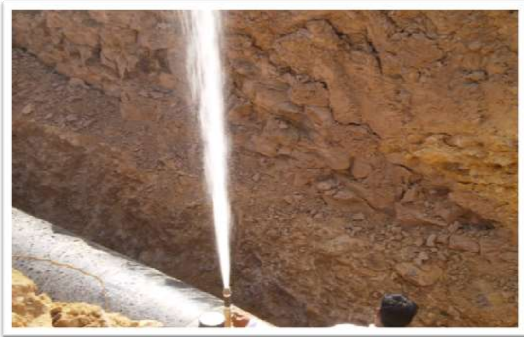
RELEASING OF PRESSURE AFTER CONDUCTING HYDROSTATIC TEST
