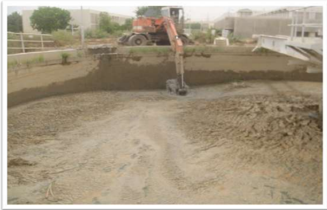
DESILTING OF POND AT NEK FILTER PLANT
