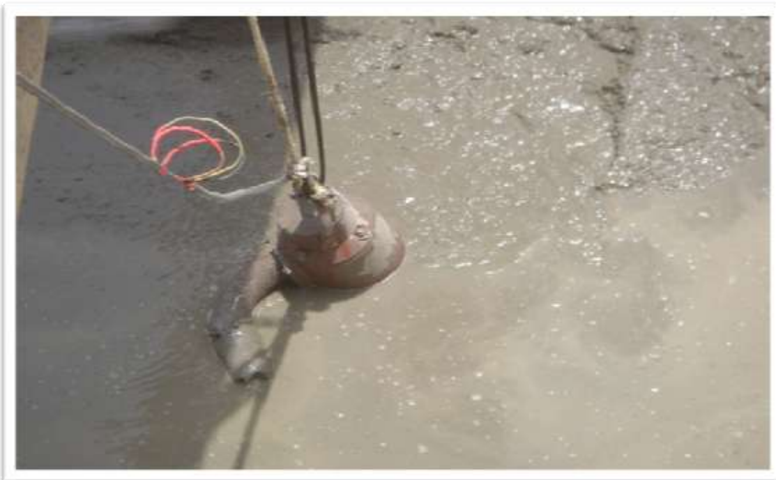
SLUSH REMOVAL IS IN PROGRESS BY SUMMERSIBLE PUMP
